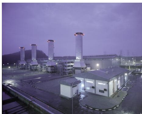
9E simple cycle gas turbines (4x123.4 MW) at Malacca, Malaysia power plant.
